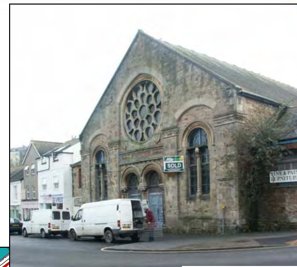
The Drill Hall
